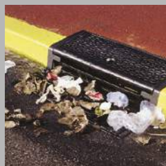
Studding on grating prevents leaves sticking to the grate and maximises flow capacity.
