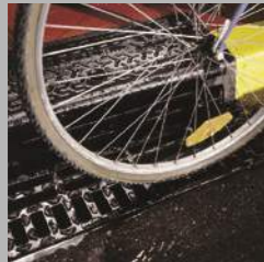
Slot orientation maximises flow capacity and road user safety.
